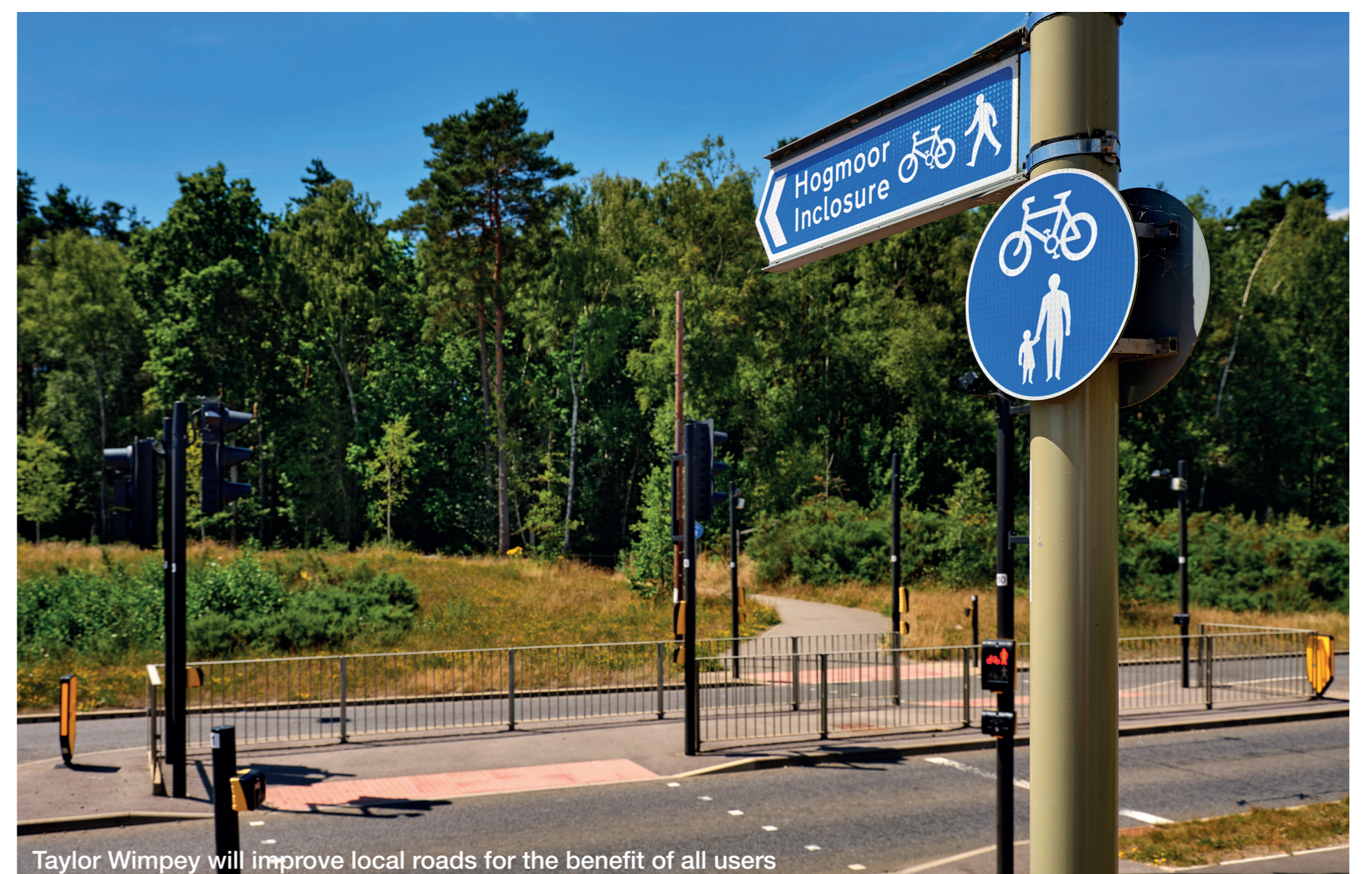
Taylor Wimpey will improve local roads for the benefit of all users
